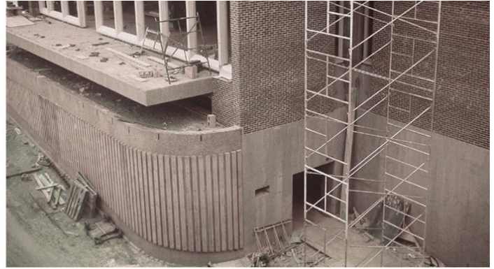
The Loading Dock Ramp - Cafeteria Above
