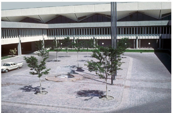
The Courtyard Completed
