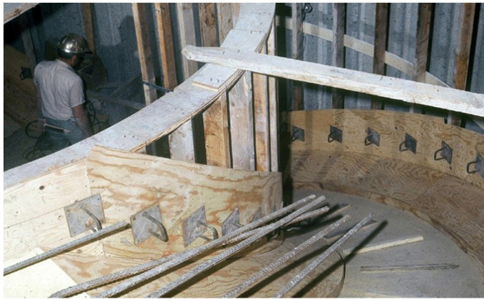
Constructing the Main Stairway
