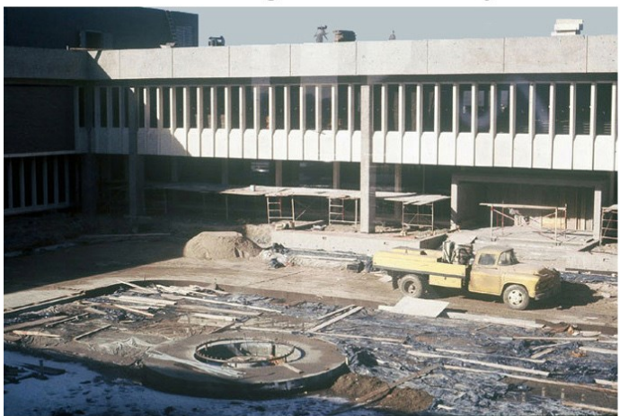
Constructing the Courtyard
