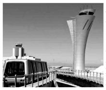
SFO and the Federal Aviation Administration (FAA) have built a new Air Traffic Control Tower that will provide the airport with the latest in technology and design. Standing 221 feet tall, the new tower features an inviting, flared design clad in curved metal paneling.
